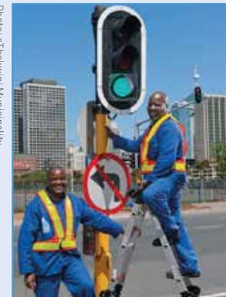
Replacing traffic lights with energy efficient LEDs
