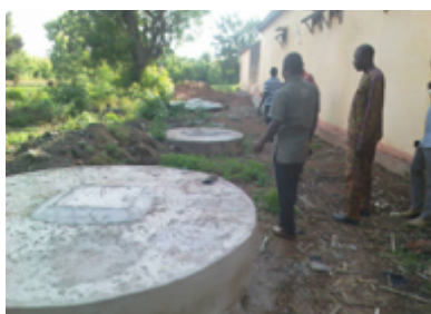
Rehabilitation of sanitary of facilities at the Mango civil prison
